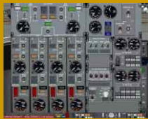
Electrical Panel designing , testing ...
